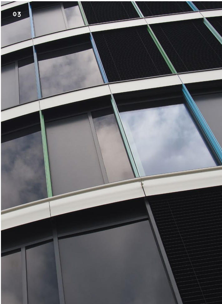
03 Blue and green shades: The façade’s special effect is created by projecting, coloured aluminium pilaster strips.
